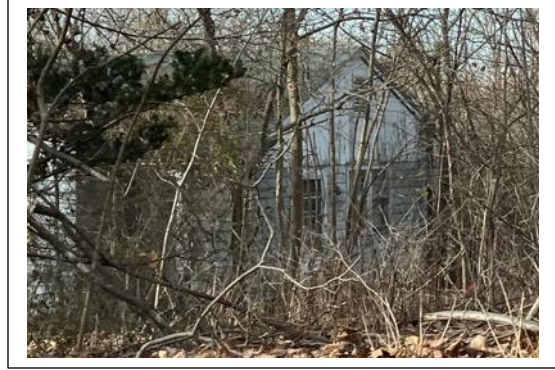
Figure 7: Neglected house ©C.M. Morawski
